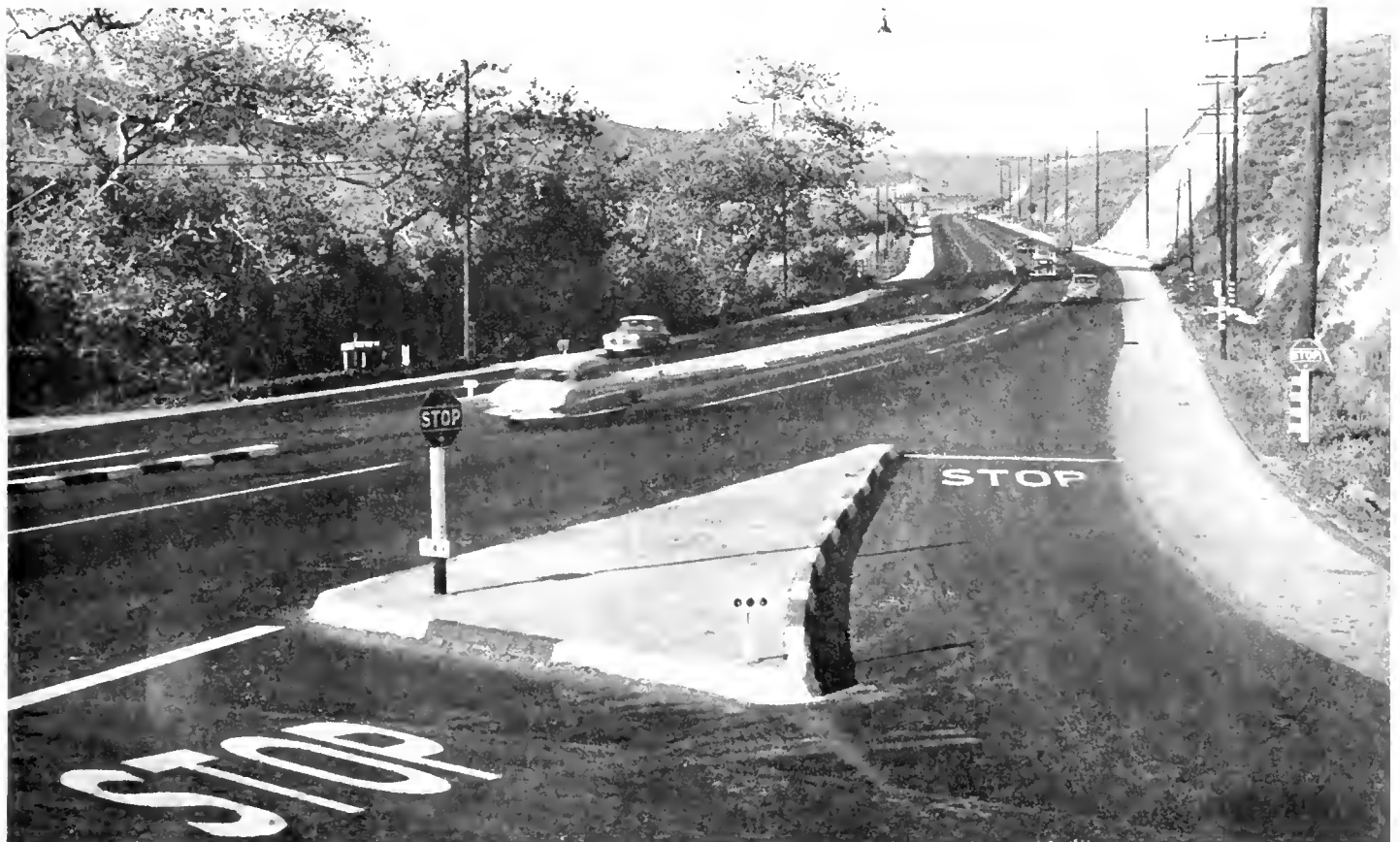
Looking northeasterly along completed construction in Zuma Canyon, showing in foreground channelization with Bonsall Drive and Westward Beach Road
